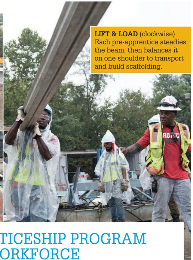
**LIFT & LOAD** (clockwise) Each pre-apprentice steadies the beam, then balances it on one shoulder to transport and build scaffolding.
